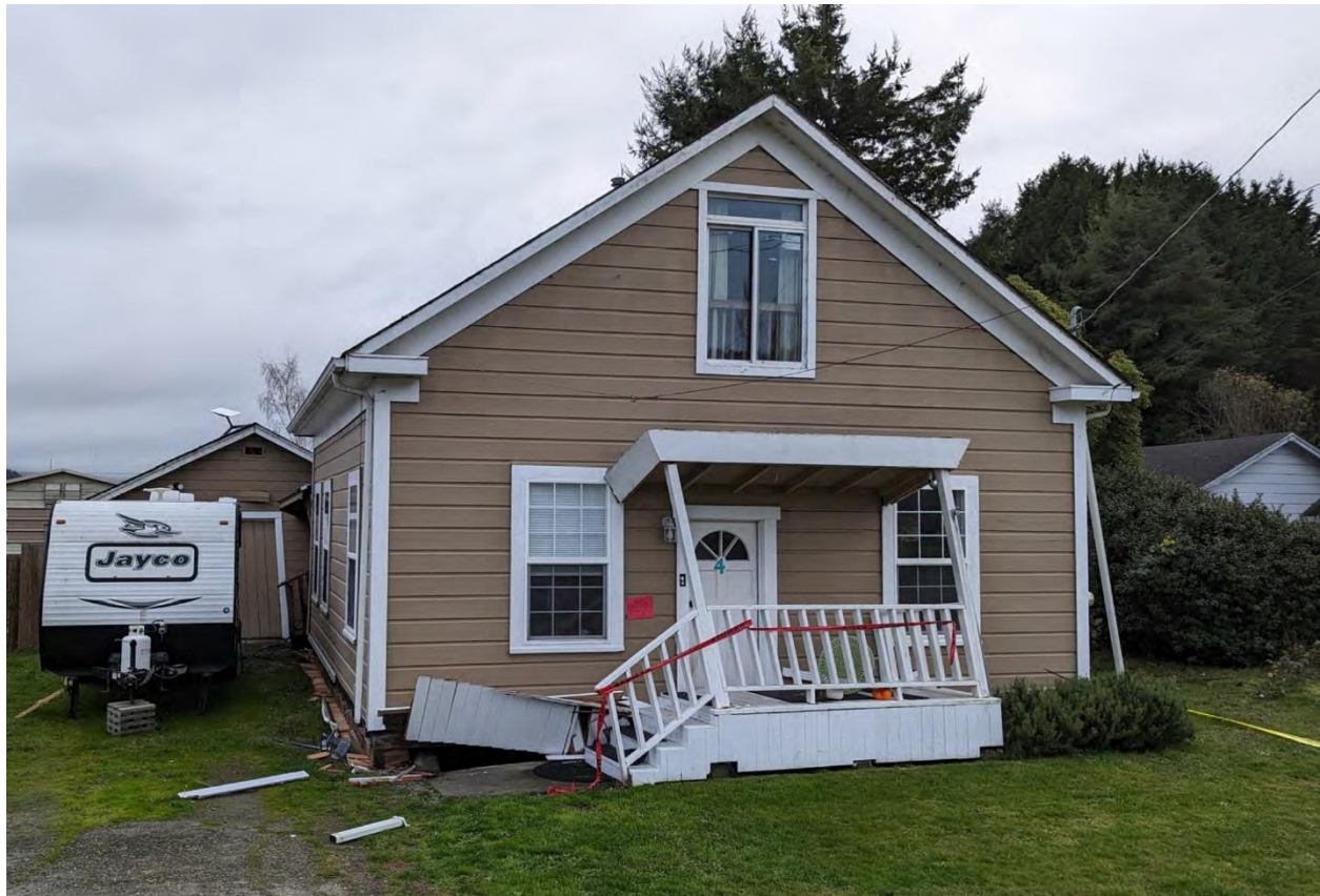
Figure 33: Earthquake Damage in Rio Dell, 2021
