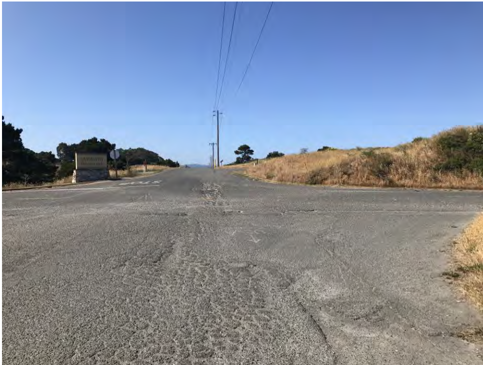
Photograph No. 8: Intersection of Vance Avenue and Bay Street.
