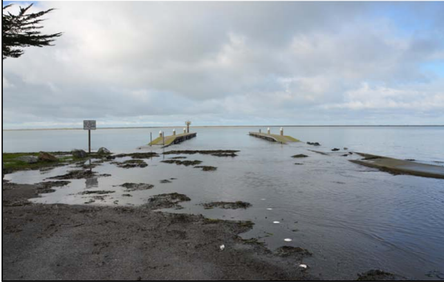
Recent nuisance saltwater flooding during a king tide in Fields Landing.
