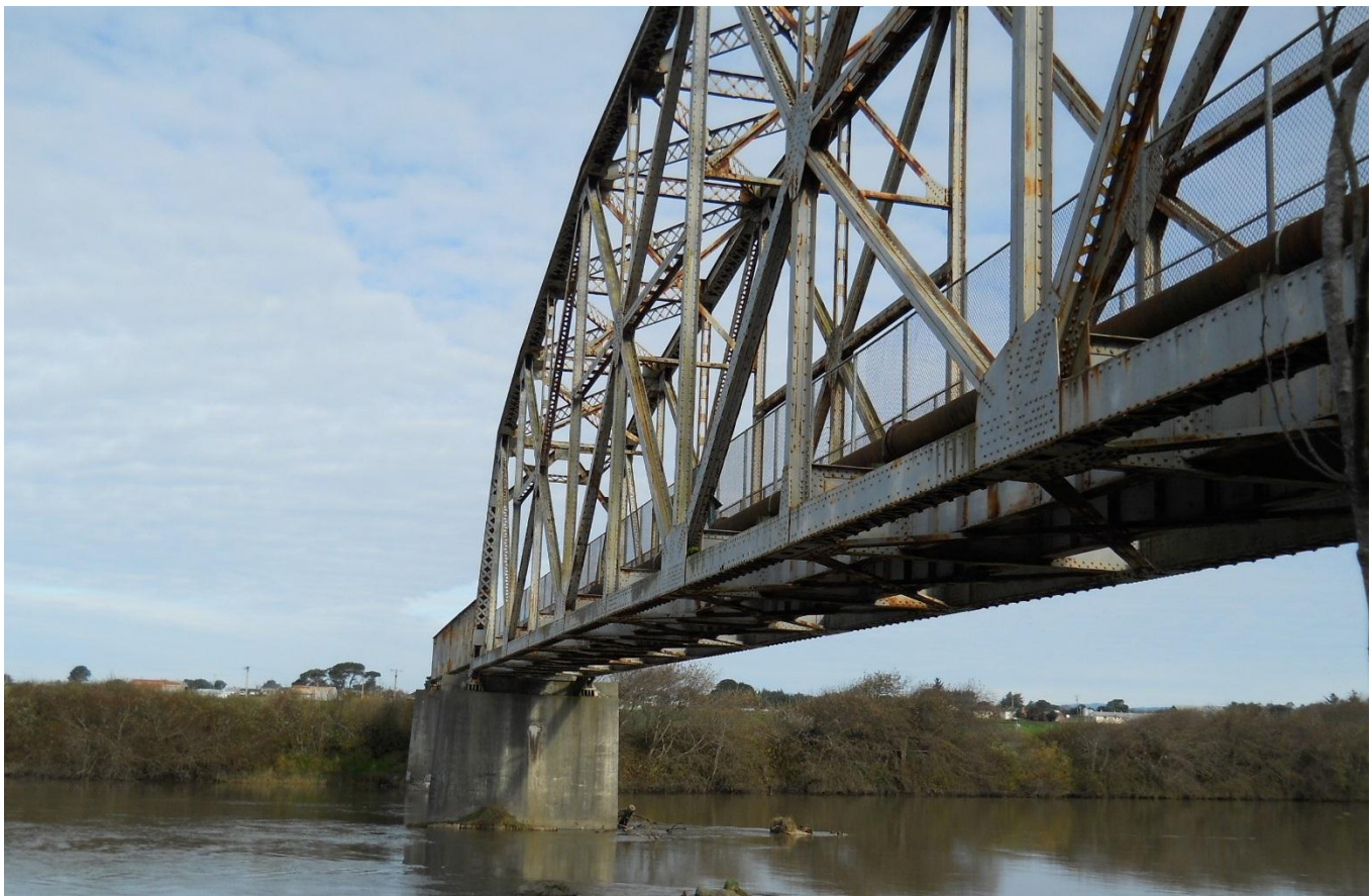
Hammond Trail Bridge over the Mad River
