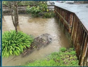
Both culverts pressurized
