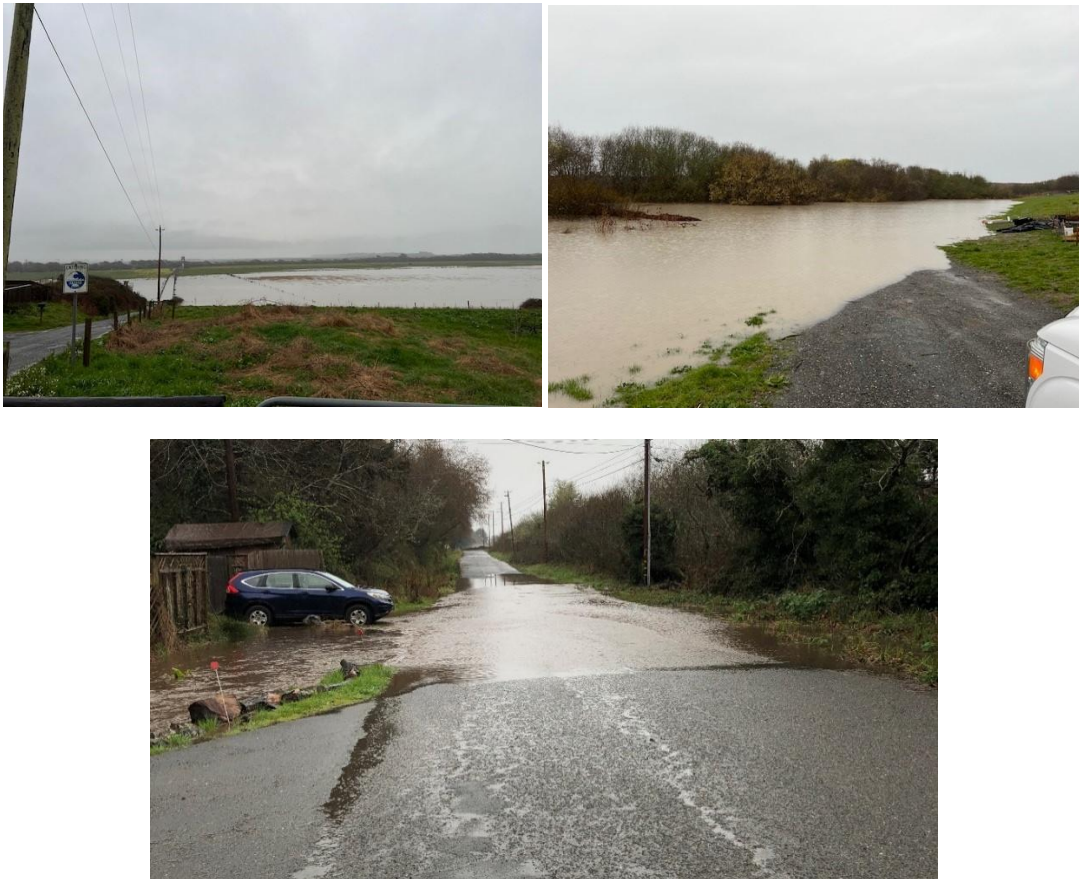
Figure 26: McKinleyville Flooding Impacts
