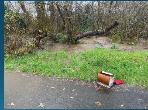
Looking upstream at potential flood retention basin
