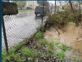
11 th Street looking west, probably 12 inches before overtopping sidewalk
