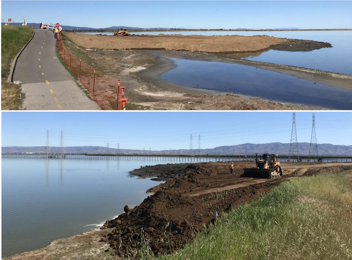
Figures 7 and 8. Direct placement of dry sediment to create a salt marsh ecotone as part of the South Bay Salt Pond Project.
