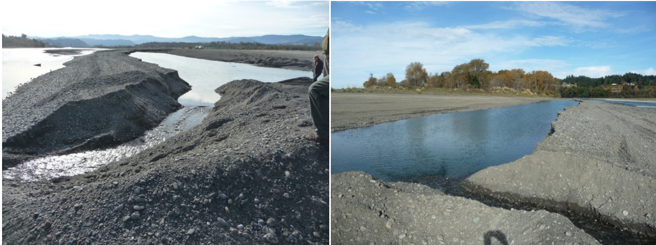
Figure 3. Trench excavated in 2013 along the Lower Eel River main channel. Left photo is at the upstream end, right is at the downstream end (photo date Nov. 6, 2013).
