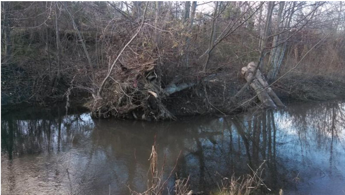
Figure 1. Habitat structures placed in lower Leggit Creek in 2012. This photo was taken in January, 2013, after high flows that occurred in December, 2012 (photo by Paul Kraus).
